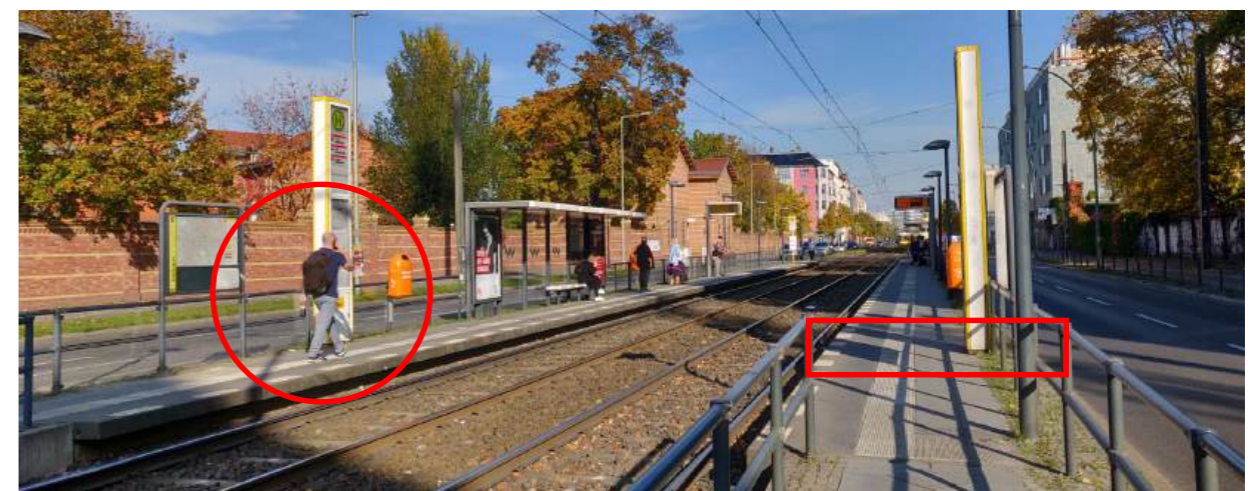
Image 3.1: A tram stop at the entrance of a major urban hospital features narrow platforms, creating challenges for wheelchair users and caregivers to access the stop and wait safely
