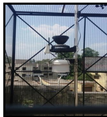
Figure 3: AWS installed at Tehsil-SADAR of Gorakhpur
