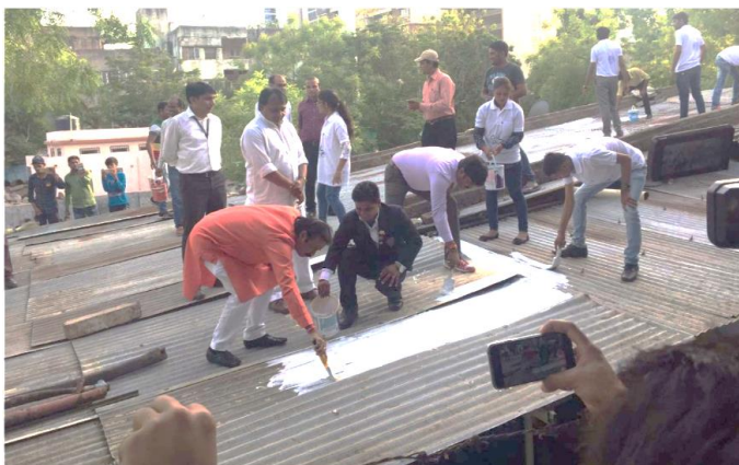
Figure 20: Ahmedabad mayor initiating cool-roof
