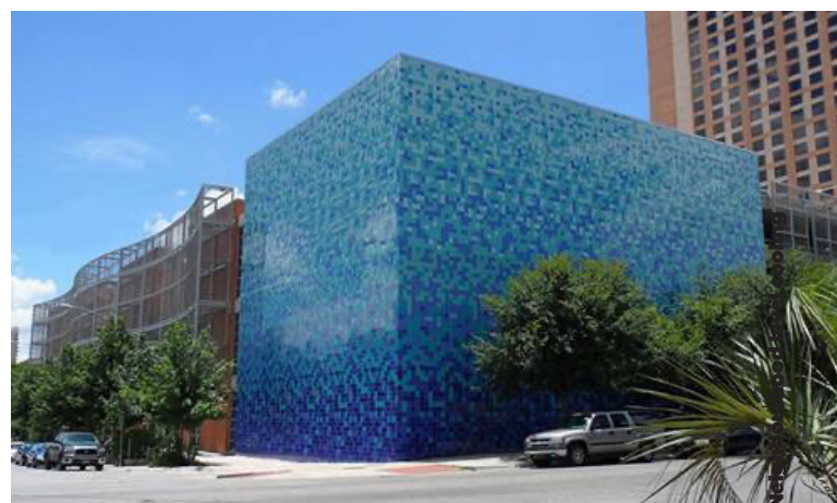
Austin Energy District Cooling Plant #2
