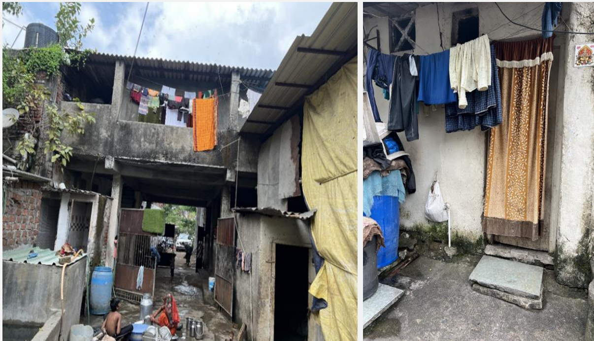
Figure: Inadequate housing infrastructure with tin roofing and no ventilation leads to increase in temperatures
