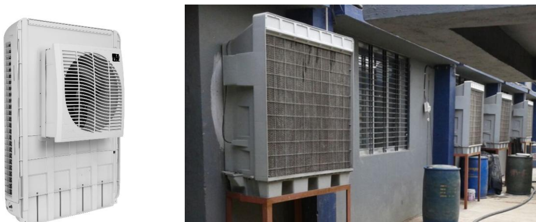
Figure 9: Examples of portable direct evaporative coolers that can be installed in a cooling center (temporary structure)
