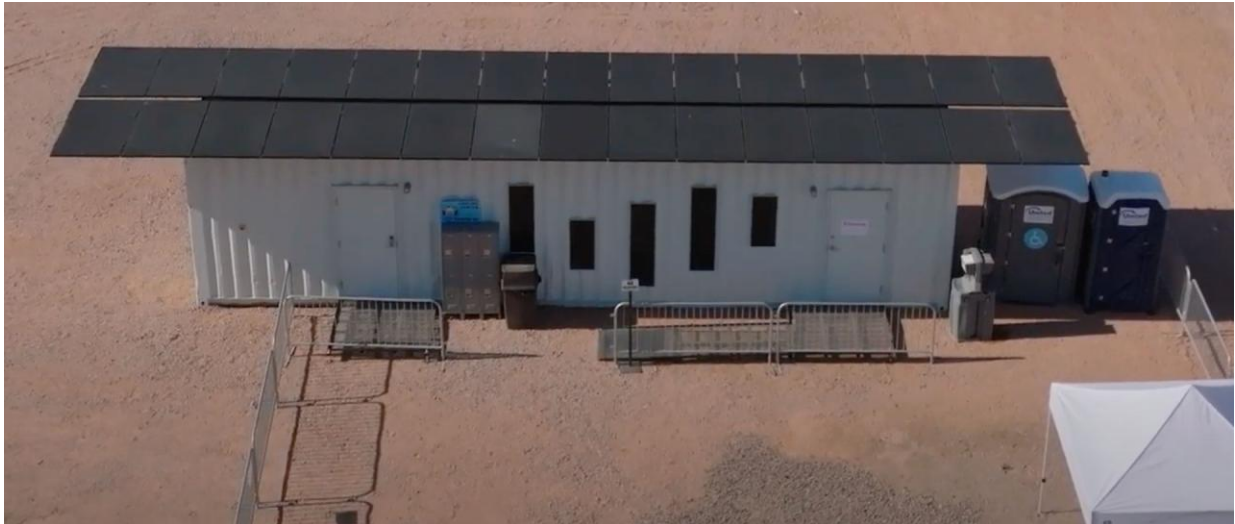
Figure 15: 'COOLtainers' located on northern Tucson's (USA) commercial corridor. These air-conditioned stations are solar-powered. One of them is equipped with cots for 5 people for napping, while the other has tables and chairs, and also offers snacks, games and hygiene items.
