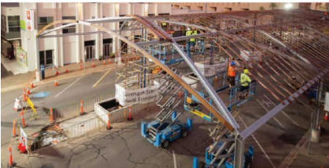
Figure 21: View of the Cavenagh Street cooling vine covered shade structure under construction in Darwin, NT. Source: Foreground
