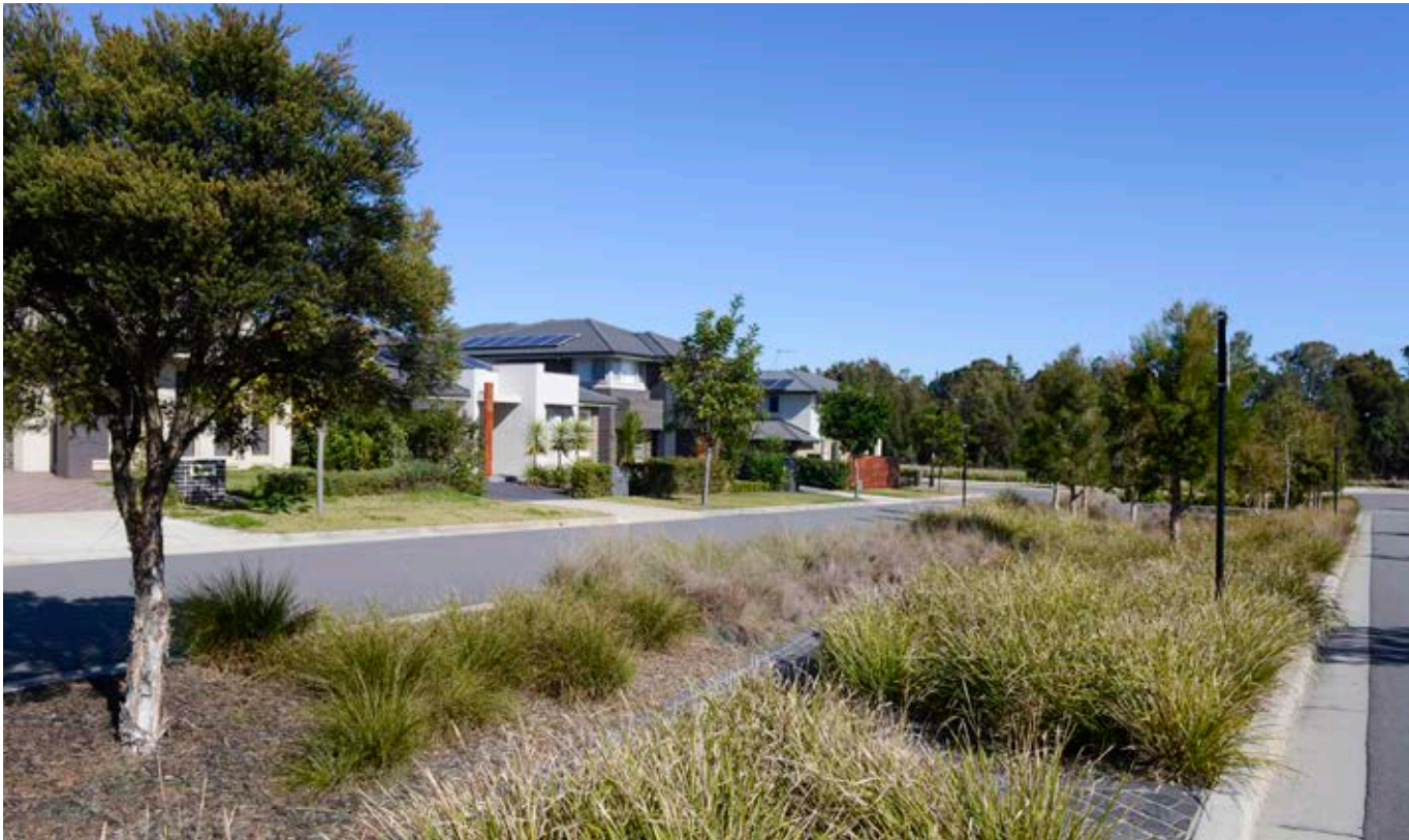
A bioswale green infrastructure project in a road median
