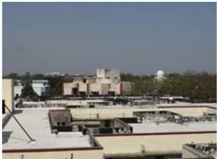
Figure 11: Shardaben General Hospital's renovated white china mosaic roof (Photo by Nehmat Kaur) 21
