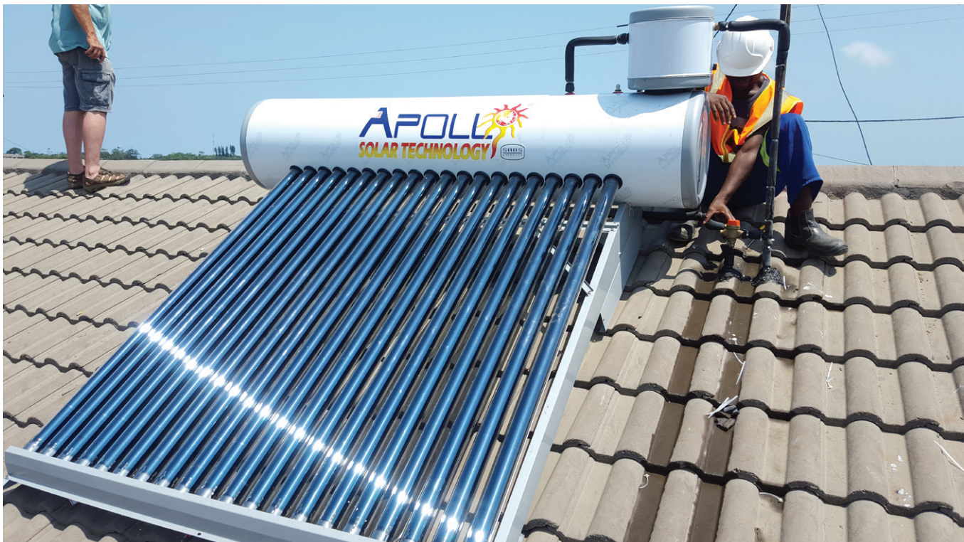
Solar water heaters save electricity and money – here installed on Groutville Care Homes in KwaDukuza, South Africa, as a pilot project implemented by Urban-LEDS
